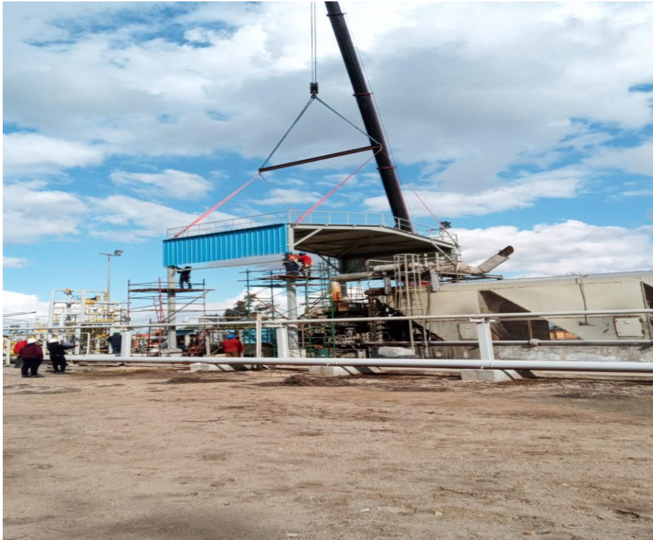
Engineering, Procurement & construction sun shed at Nodal area Contract No : (PR-545)
