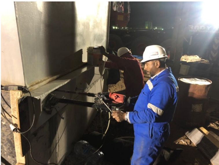
knock out drum replacement
